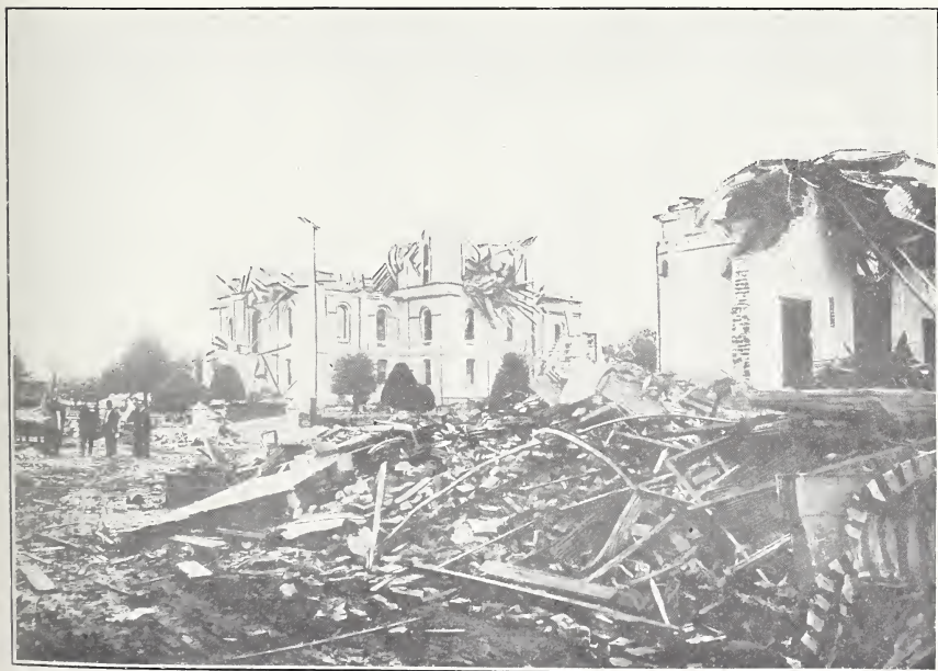
B. COMPLETE WRECK BY EARTHQUAKE, COURT-HOUSE AND HALL OF RECORDS, SANTA ROSA.
